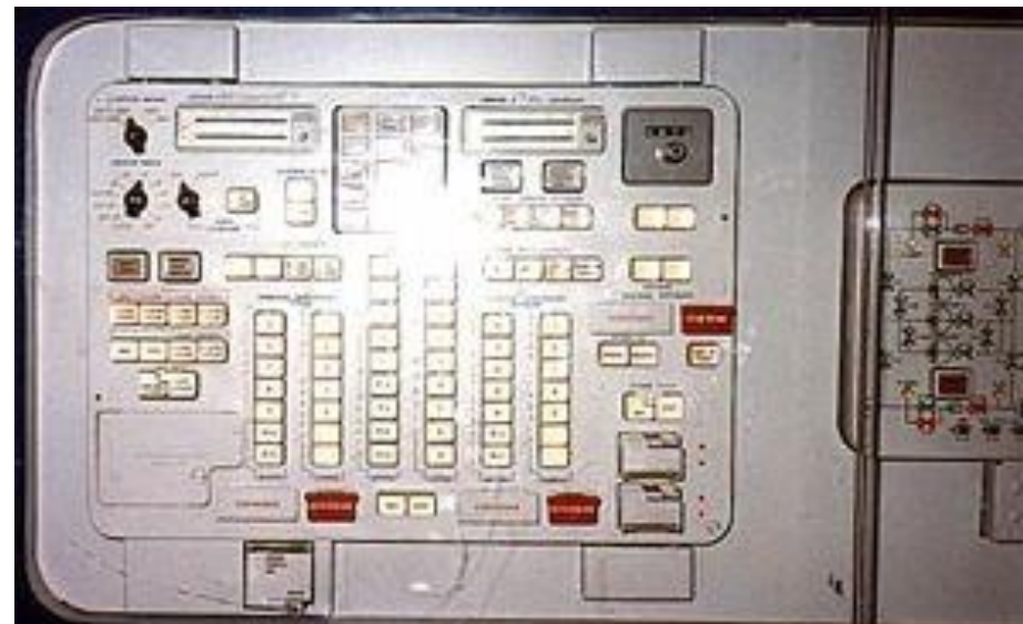
Propellant control system panel
